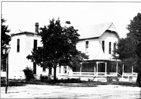
RESIDENCE OF MRS. CLELAND.
